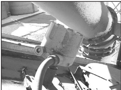
This installed KA unit is being used as a high-level alarm in a grain storage application.
